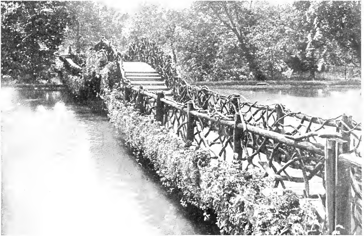
A rustic bridge with steps to overcome the slight rise of the arch in the centre span.
